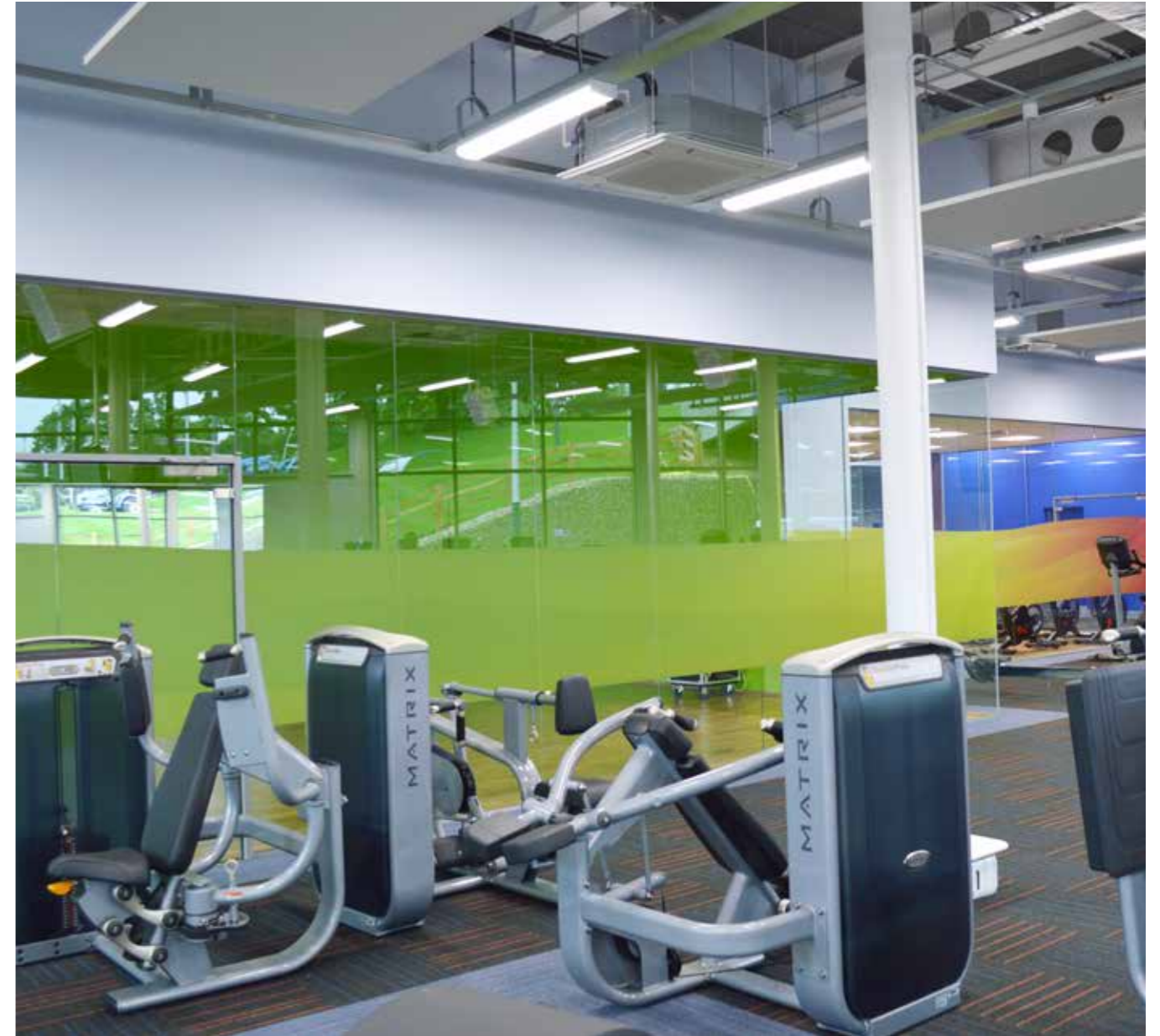
Subtle blended gradients printed to dusted vinyl to meet DDA requirements and add privacy for gym users.
