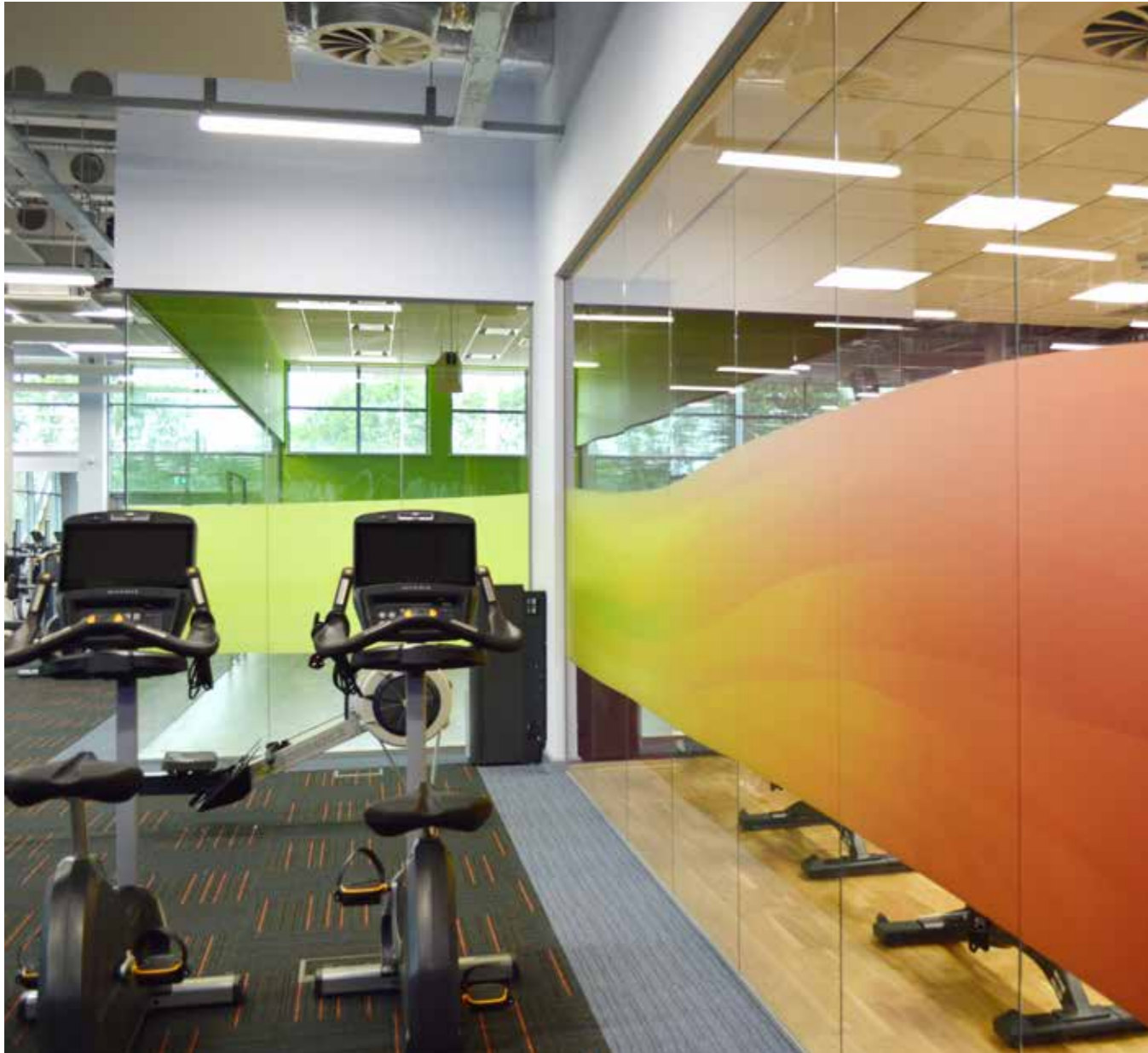
Printed dusted window vinyl to create privacy for the spin classes and fitness studio,. Colours were used to match the existing wall colours and we blended them to create a gradient of colour.
