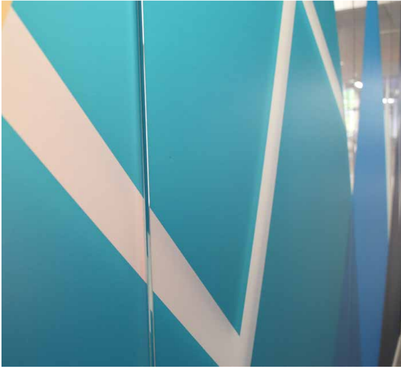
Printed dusted window film was cut to shape in a mountain formation to allow light into the room and maintain low-level privacy for climbers
