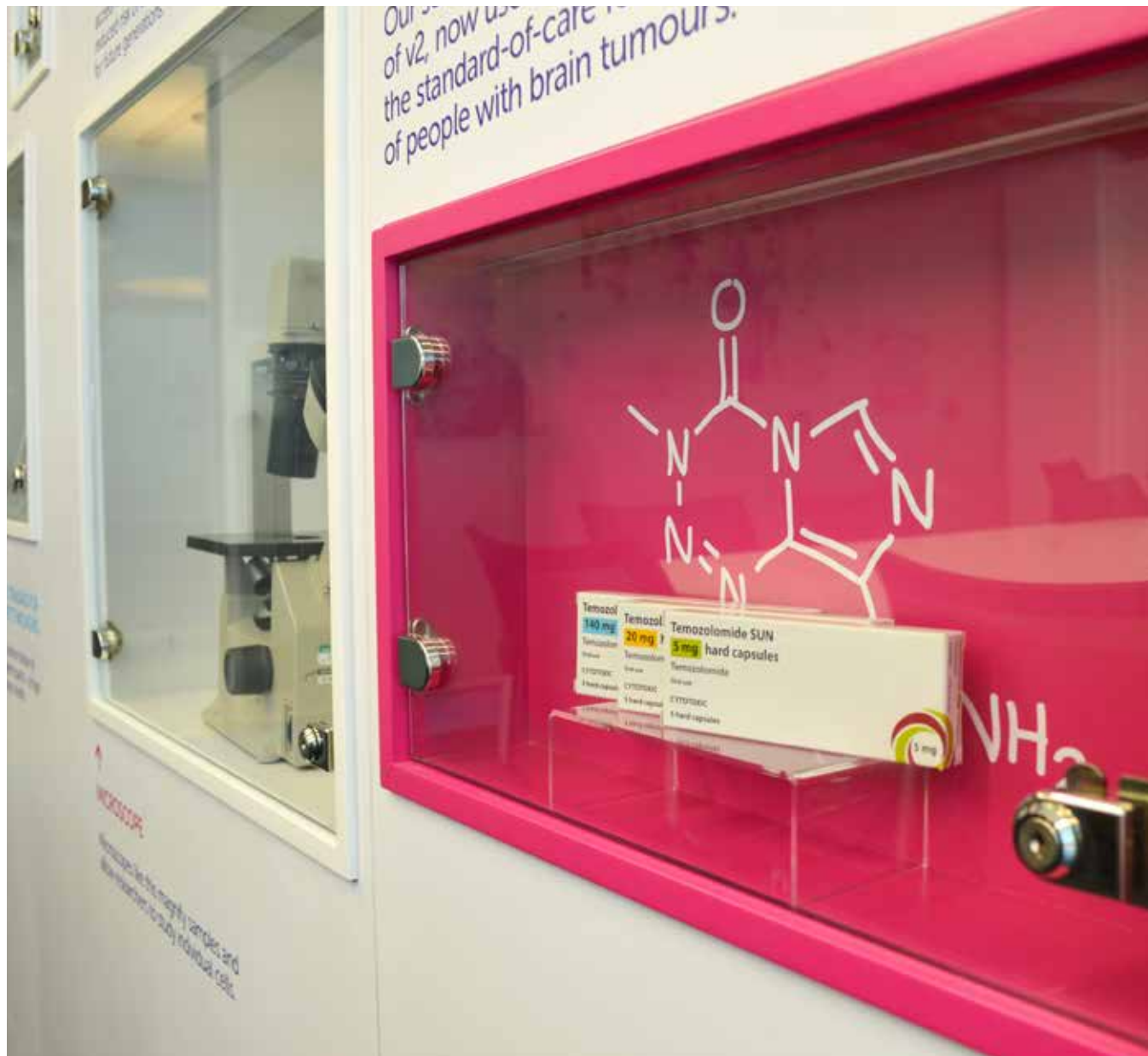
Hinged and lockable glass doors with colour coordinated vinyl graphics applied to the back of the recess.
